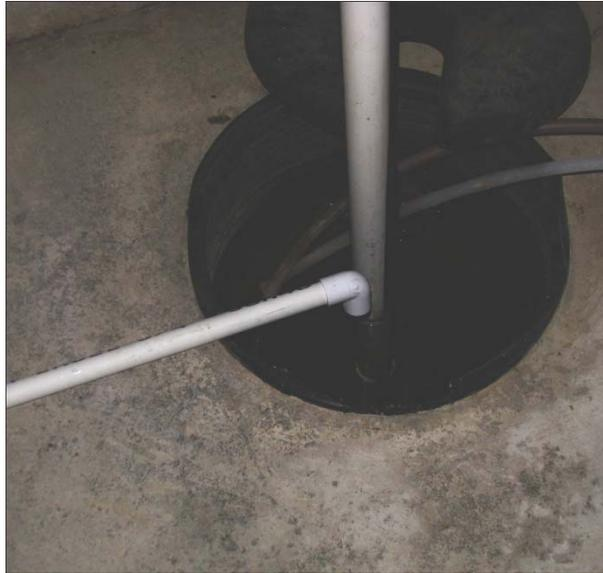
**Drain from power heads to the sump pump housing**
